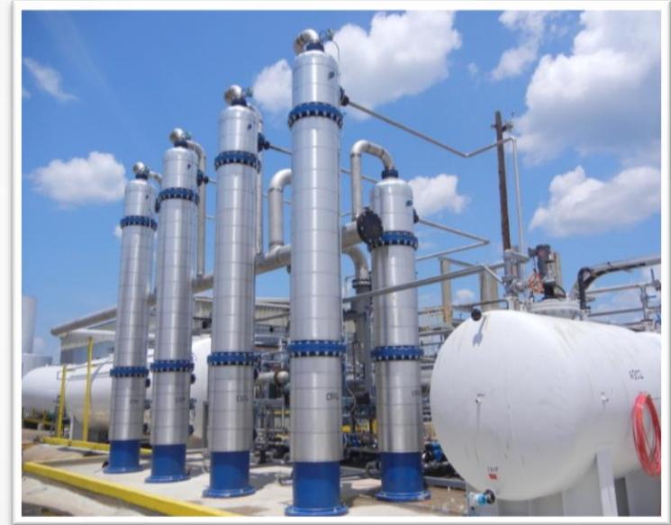
Esterification system at Vanguard Biodiesel, Louisiana
